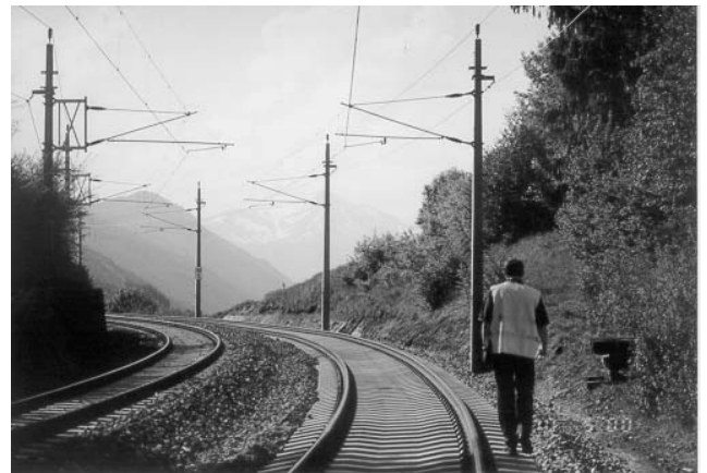
Figure 14 General view of test site, ÖBB system
