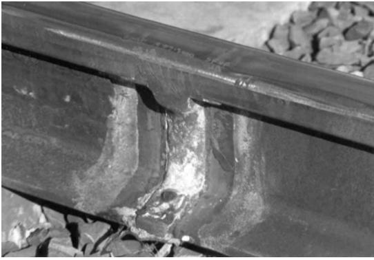
Figure 11 General view of 2-component weld in 68 kg/m rail
