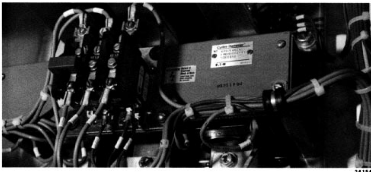
Figure 4. Typical Overload Relay
