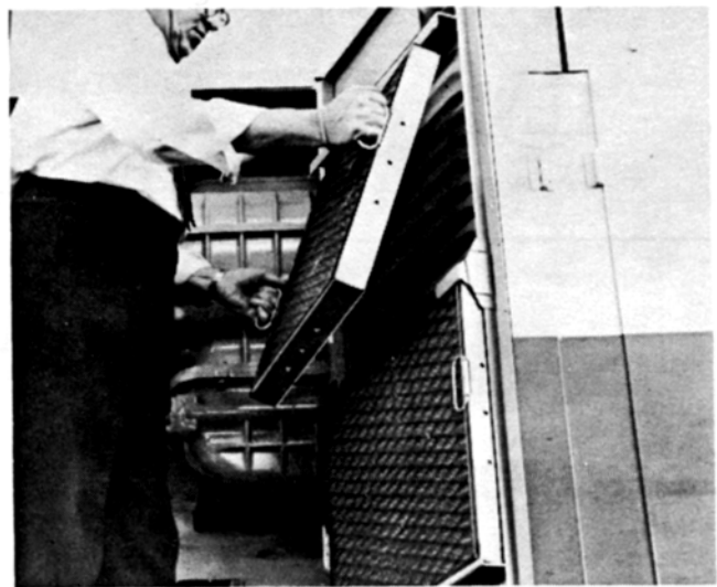
Fig. 3 - Removal Of Filters
