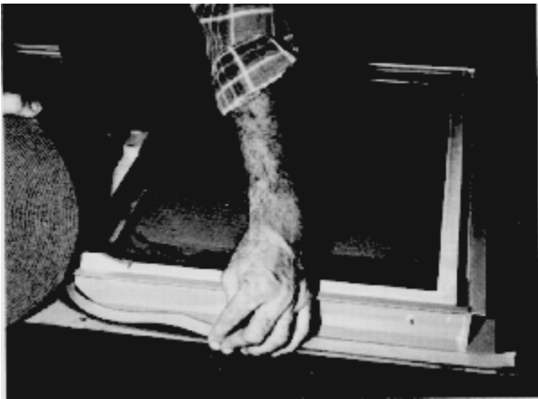
Fig. 13 - Plastic Tape Application To Back Side
