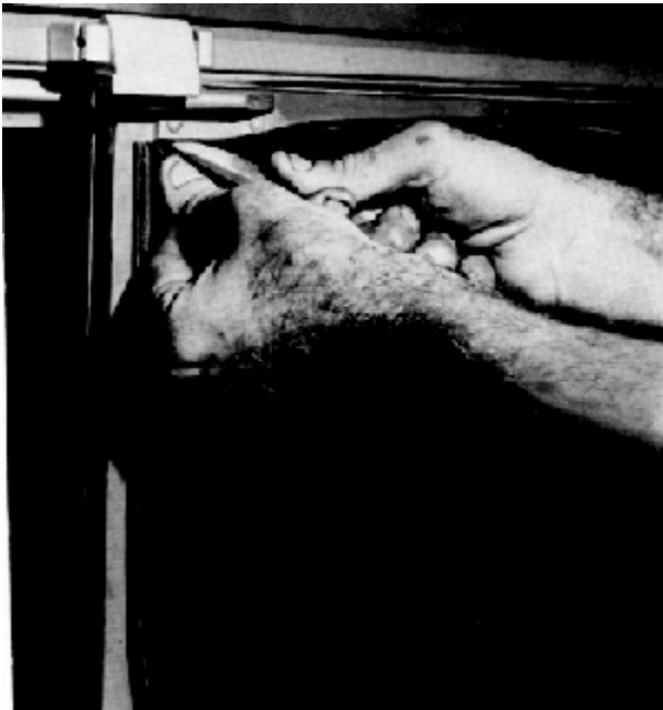
Fig. 16 - Mated Corners Being Inserted Into Glass Track With Bone Stick
