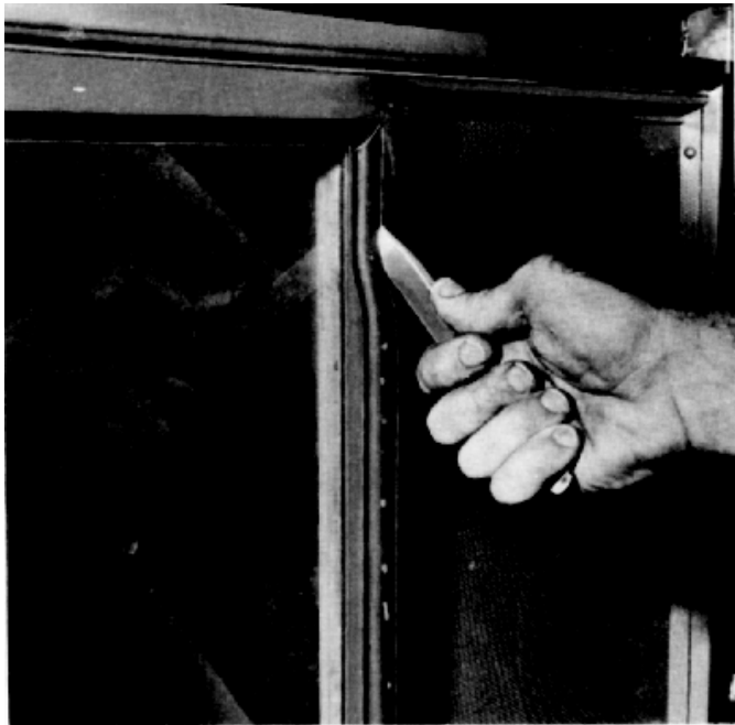
Fig. 18 - Corners Completed - Zipper-Like Bone Stick Motion Completes Glazing Strip Installation
