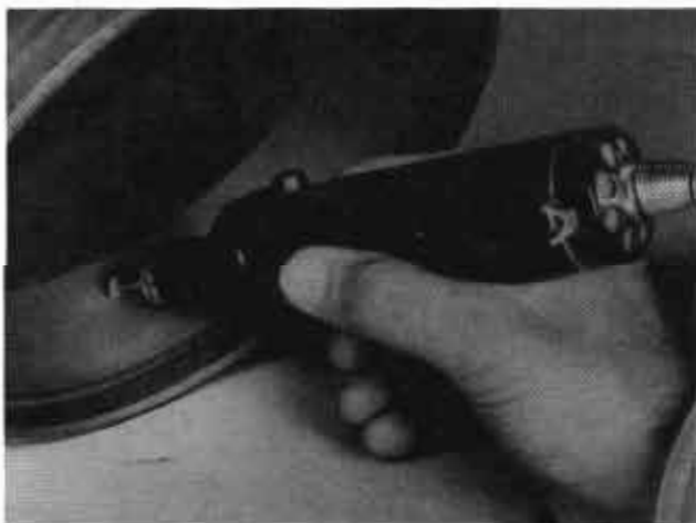
Grinding Spall With Pencil Grinder
