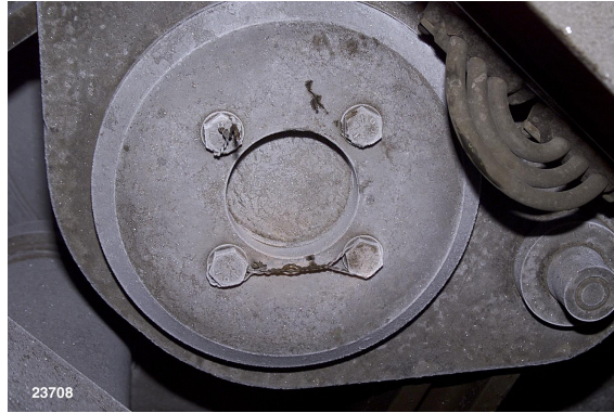
Figure 26 – Lock Wire and Bolt Removal
