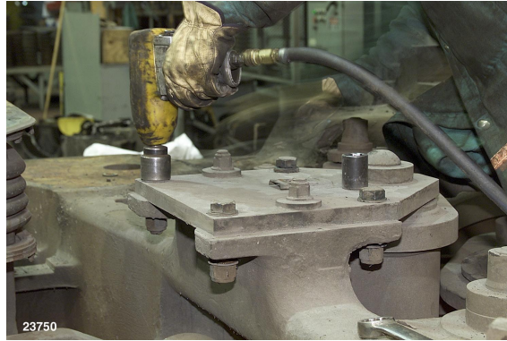
Figure 36 – Removing Plate Bolts
