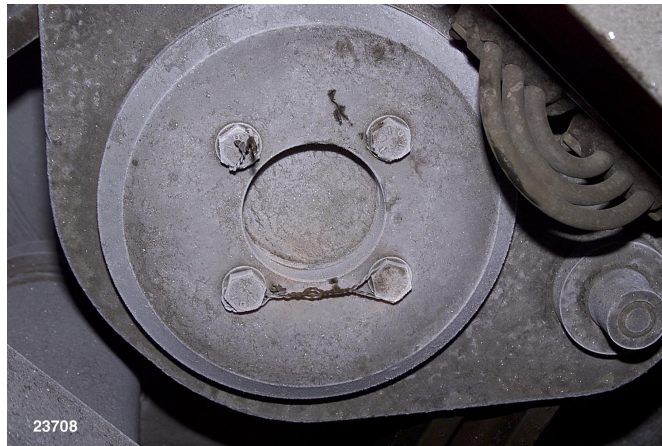
Figure 32 – Application of Safety Wire
